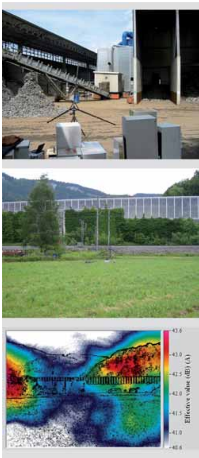
Figure 3: Waste separation plant and photos of noise exposure ((c) GFal)
