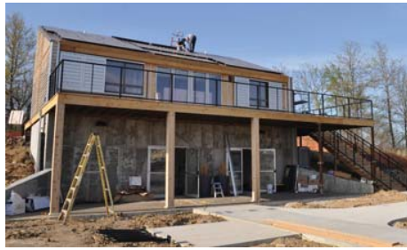
The repurposed ISU Solar Decathlon House under reconstruction at Honey Creek.
